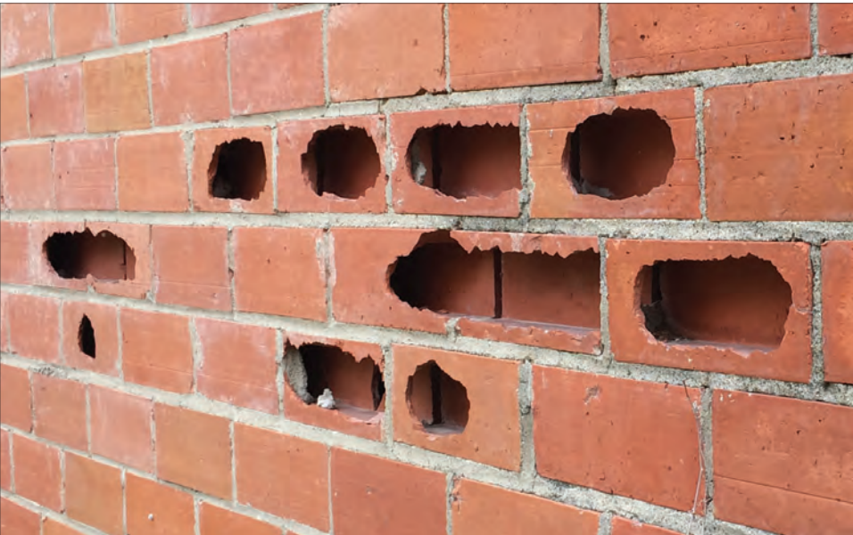
Brick damage at rear of building should be carefully repaired.
