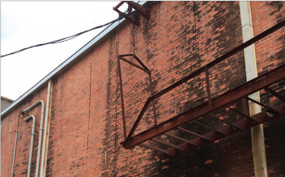
Current state of rear of theater. Careful cleaning of brick is needed.
