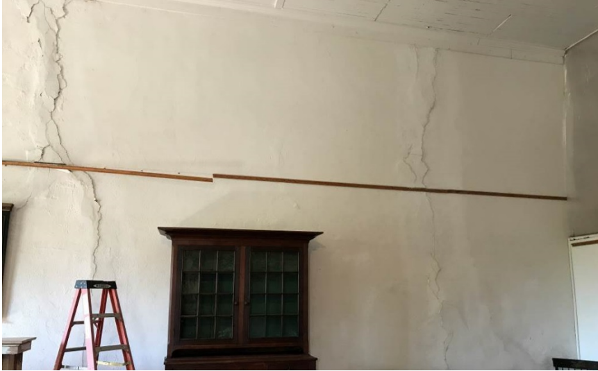
View of plaster walls showing large cracks from floor to ceiling, Oct. 2017
