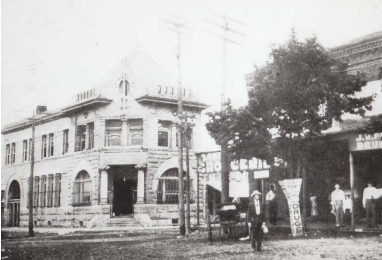
View of Farmers and Merchants Bank Building from the southeast, 1910
