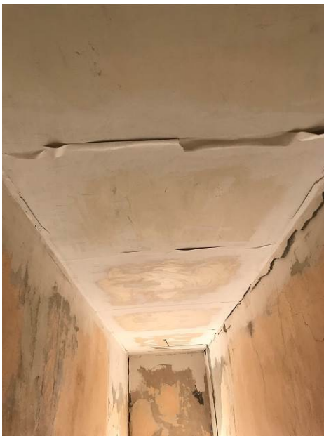
Sheetrock ceiling in stairway to second floor, Oct. 2017
