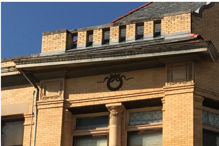
Pressed metal projecting cornice, Oct. 2017
