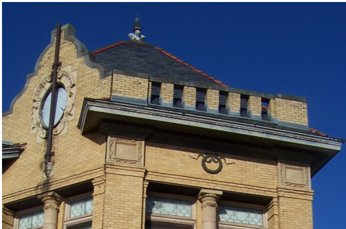
Square hipped gray slate roof, Oct. 2017
