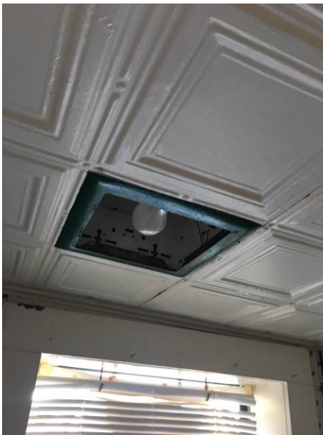
Coffered metal tin ceiling in the second floor bathroom, Oct. 2017
