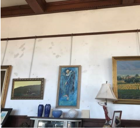
Plaster walls with unmatched paint touchups and cracks above windows and doors, Oct. 2017
