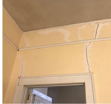
Plaster walls with unmatched paint touchups and cracks above windows and doors, Oct. 2017
