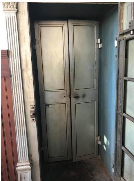
Inner vault metal doors, Oct. 2017
