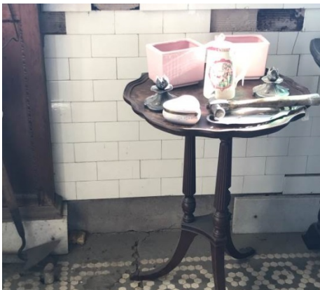
Marble wall base in the lobby, Oct. 2017
