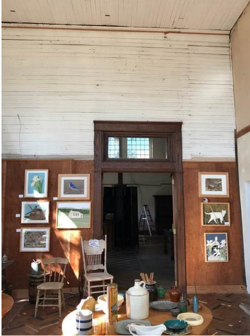
Beadboard and plywood ½ wall, Oct. 2017
