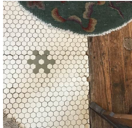
Tile pattern with visible large cracks and showing where the tile meets the stained wood floor, Oct. 2017
