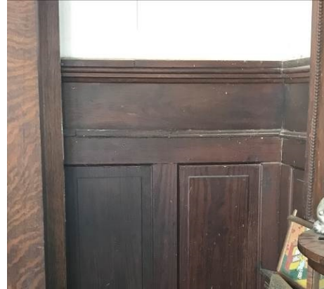
Wood panel wainscoting in lobby, Oct. 2017
