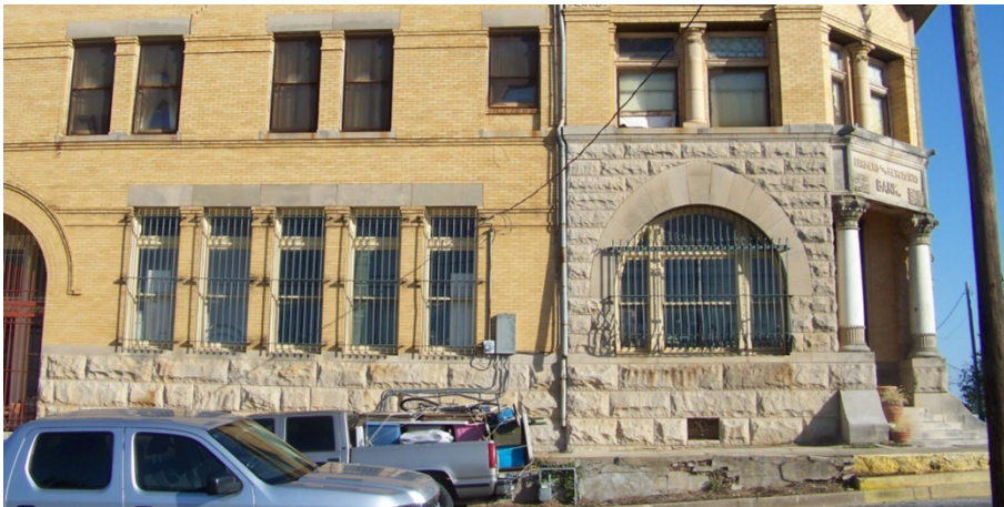
Rusticated limestone water table and entrance porch, Oct. 2017
