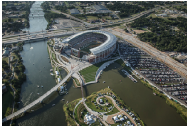
McClane Stadium Across the Riverwalk (0.5 miles)
