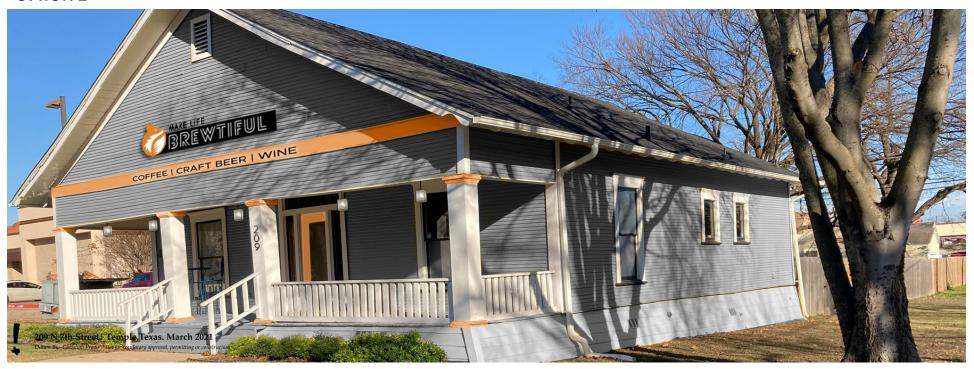
Proposed neon signage can be mounted on a backing frame pinned through exterior wall. The wall studs might not align with the position of the pins. It is also important the use of sealant where the pins penetrate the wall surface. This will prevent moisture from entering the wall and deteriorating the framing members. Refer to sketch at the end of the report for south facade mural proposal.
