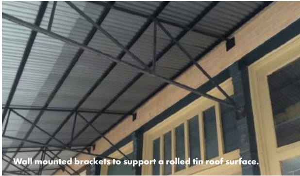
Rolled tin roof surface
