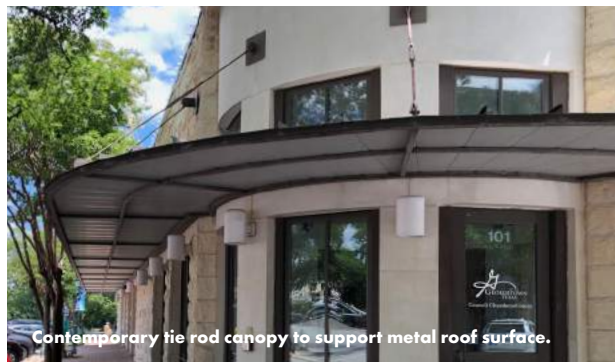
Contemporary tie rod canopy with wood soffit.
