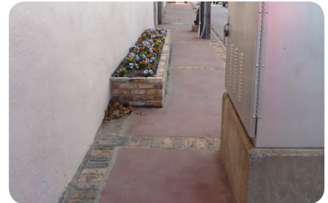
Above/Below: Modifications, such as the ones shown, are not compliant per the 2012 Texas Accessibility Standards. For example, the image above shows the addition of a ramp without considering the required slope or barrier edge protection.
