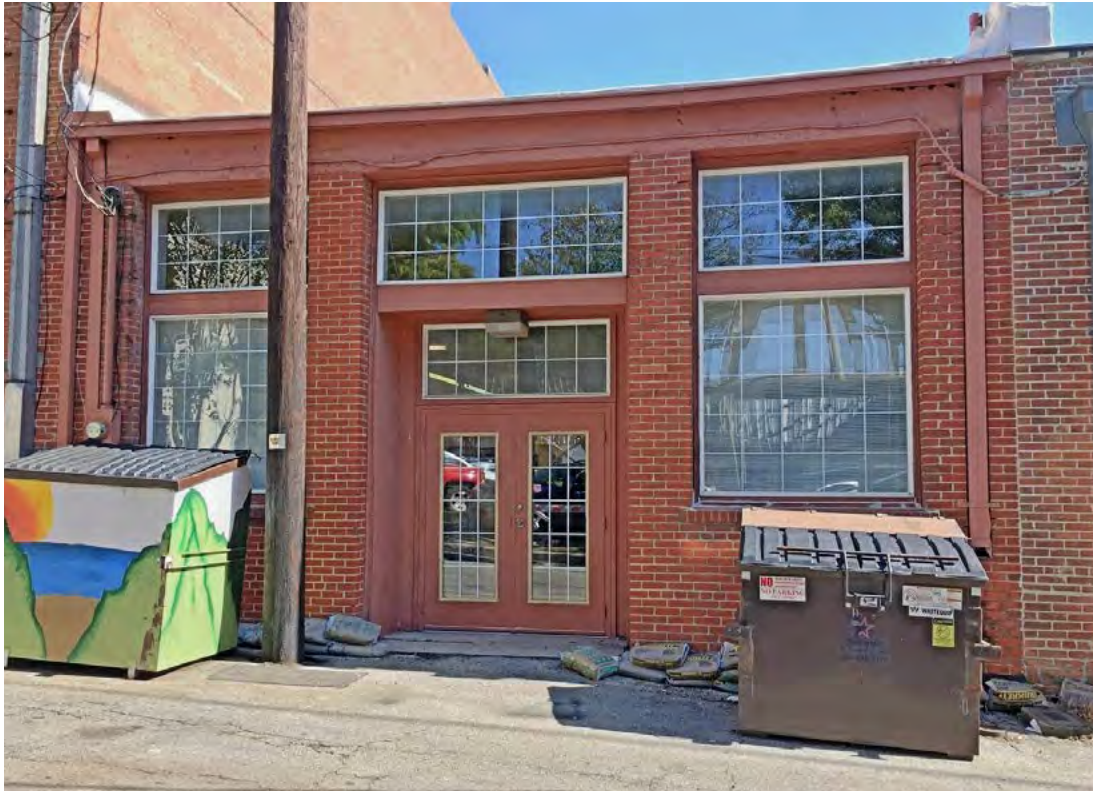
EXISTING - REAR FACADE
