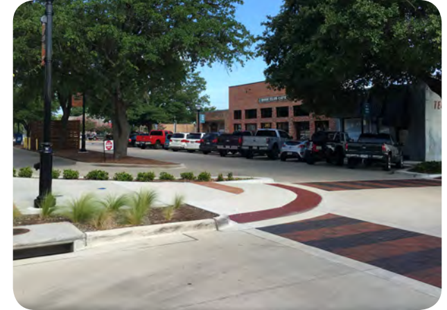
2. Durable Liquid Pavement Markings, including epoxies and resins, is a durable, economical approach that requires special equipment for application and has a life span of 3 to 6 years.
