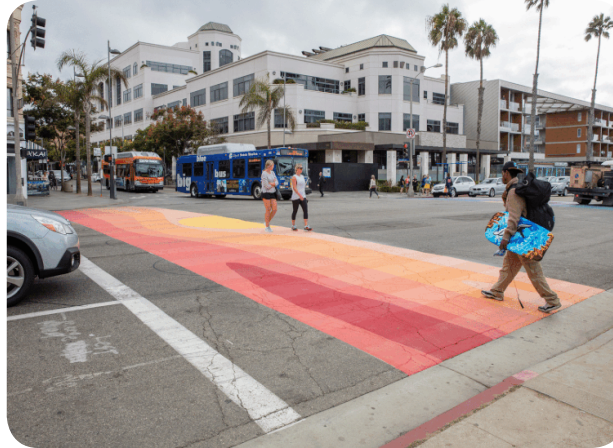
1. Paint is the most commonly used method, yet is considered a non-durable pavement marking due to an expected lifespan of 6 months to 2 years. Paint can be applied in many ways, including sprayers and rollers, making it more accessible for volunteers. (Untitled, Santa Monica, CA. Artist: Here LA)
