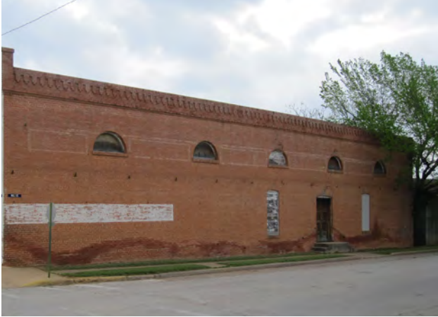
Rising Damp: Excessive moisture in the ground, crawl space, or basement is visible on wall surfaces, as the brick appears visibly darker when damp (above left). Moisture causes brick deterioration (above right). Additional drainage around the building or drying of interior spaces is needed.
