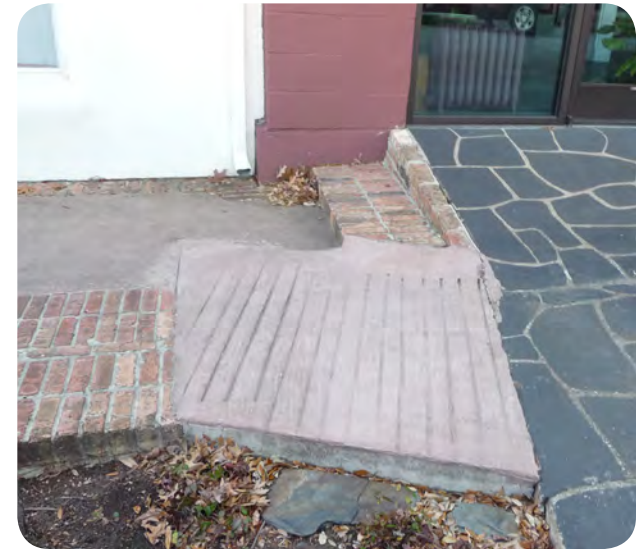
Above/Below: Modifications, such as the ones shown, are not compliant per the 2012 Texas Accessibility Standards. For example, the image above shows the addition of a ramp without considering the required slope or barrier edge protection.
