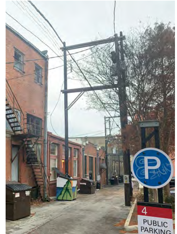
EXISTING - REAR FACADE
