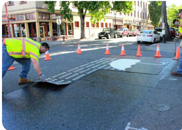
3. Thermoplastic can be applied as a liquid through spraying from specialized equipment or in sheets that are heated in place to create a single surface. The average lifespan is 5 years.
