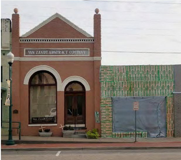
Above: Van Zandt Abstract Company in Canton, Texas carefully removed layers of paint from their front facade using Dumond Peel Away Poulitice system. Below: This process revealed the natural color of the brick and a ghost sign.
