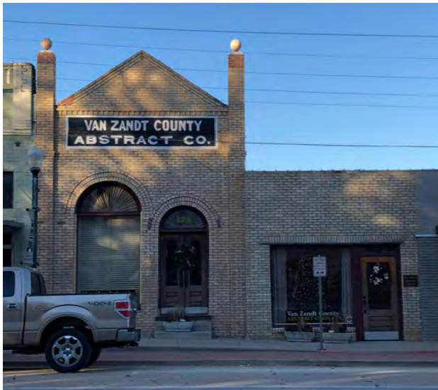
Above: Van Zandt Abstract Company in Canton, Texas carefully removed layers of paint from their front facade using Dumond Peel Away Poulitice system. Below: This process revealed the natural color of the brick and a ghost sign.
