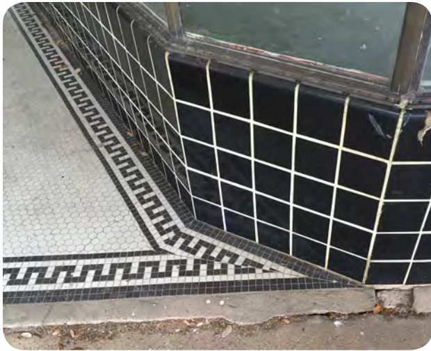
Above: Corsicana, Texas. Historic materials, such as this mosaic tile on Corsicana's Beaton Street within a recessed entry, should be carefully preserved during sidewalk repair or construction. Below: Another type of extension is a 'bus bulb', where the sidewalk extends to 1 to 2 feet of the parking lane to create space for the bus stop.
