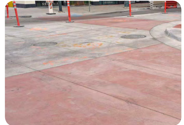
4. Colored pavement, including asphalt and concrete, utilizes colored pigment within the material mix. For asphalt, the pigment is mixed into a thin layer on the surface. For concrete, pigment is added to the concrete mix, with color going all the way through ensuring color will not fade or chip.
