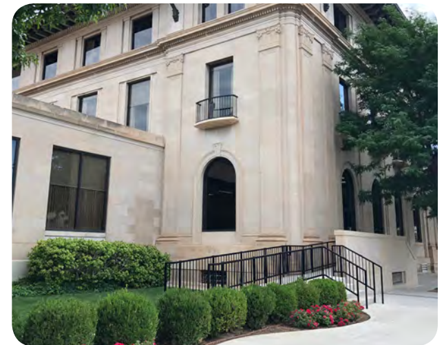
Above: Bistro 108, La Grange, Texas. The image above demonstrates the modification to an existing building entry in order to provide an accessible route for restaurant guests and employees. Below: Amarillo, Texas. Access from the sidewalk to the building are one component of an 'accessible route'.
