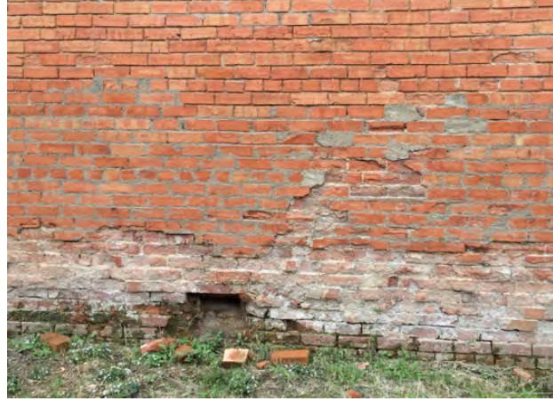
Rising Damp: Excessive moisture in the ground, crawl space, or basement is visible on wall surfaces, as the brick appears visibly darker when damp (above left). Moisture causes brick deterioration (above right). Additional drainage around the building or drying of interior spaces is needed.
