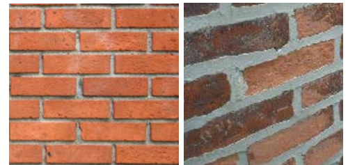
Recessed Joints vs. Flush Joints
