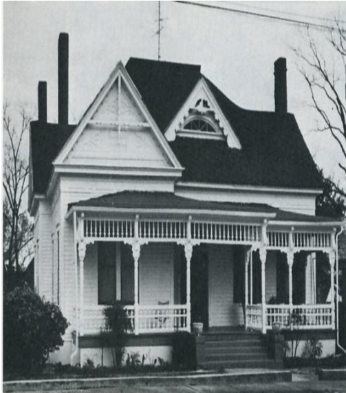
(Left) Queen Anne Style: Note the spindlework, unique dormers, and detailed porch columns.
