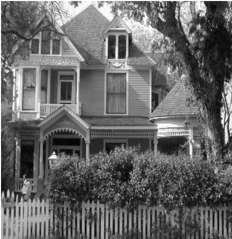
(Left) Wood windows should be retained if at all possible. This Queen Anne has retained the wood windows but has replaced the panes with a single pane instead of a multiple pane.
