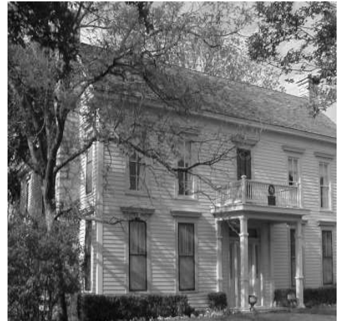
(Left) Wood windows should be retained if at all possible. This Queen Anne has retained the wood windows but has replaced the panes with a single pane instead of a multiple pane.
