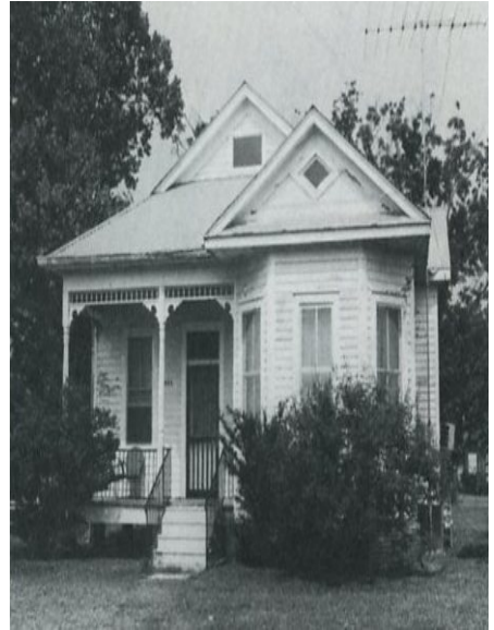
(Right) Much simpler example. Corner bracket detailing is missing Spindles and and porch column details are still present.
