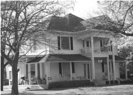
(Right) Front porch has been converted into sun room. Construction has been consistent with architectural features but has diminished the historical character of the structure.
