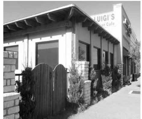
(Left) Variety in parapet detail adds character. Mansard roof should be returned to original construction
