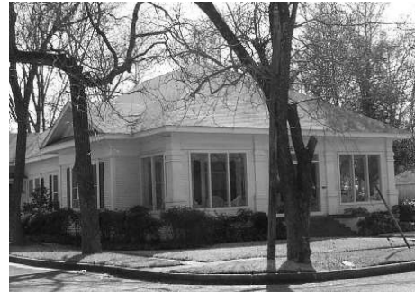
(Right) Front porch has been converted into sun room. Construction has been consistent with architectural features but has diminished the historical character of the structure.
