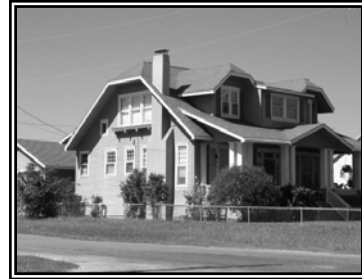
Clipped Gable Roof
