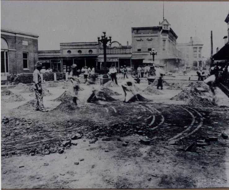
Figure 20: Taking up blocks and paving the square
