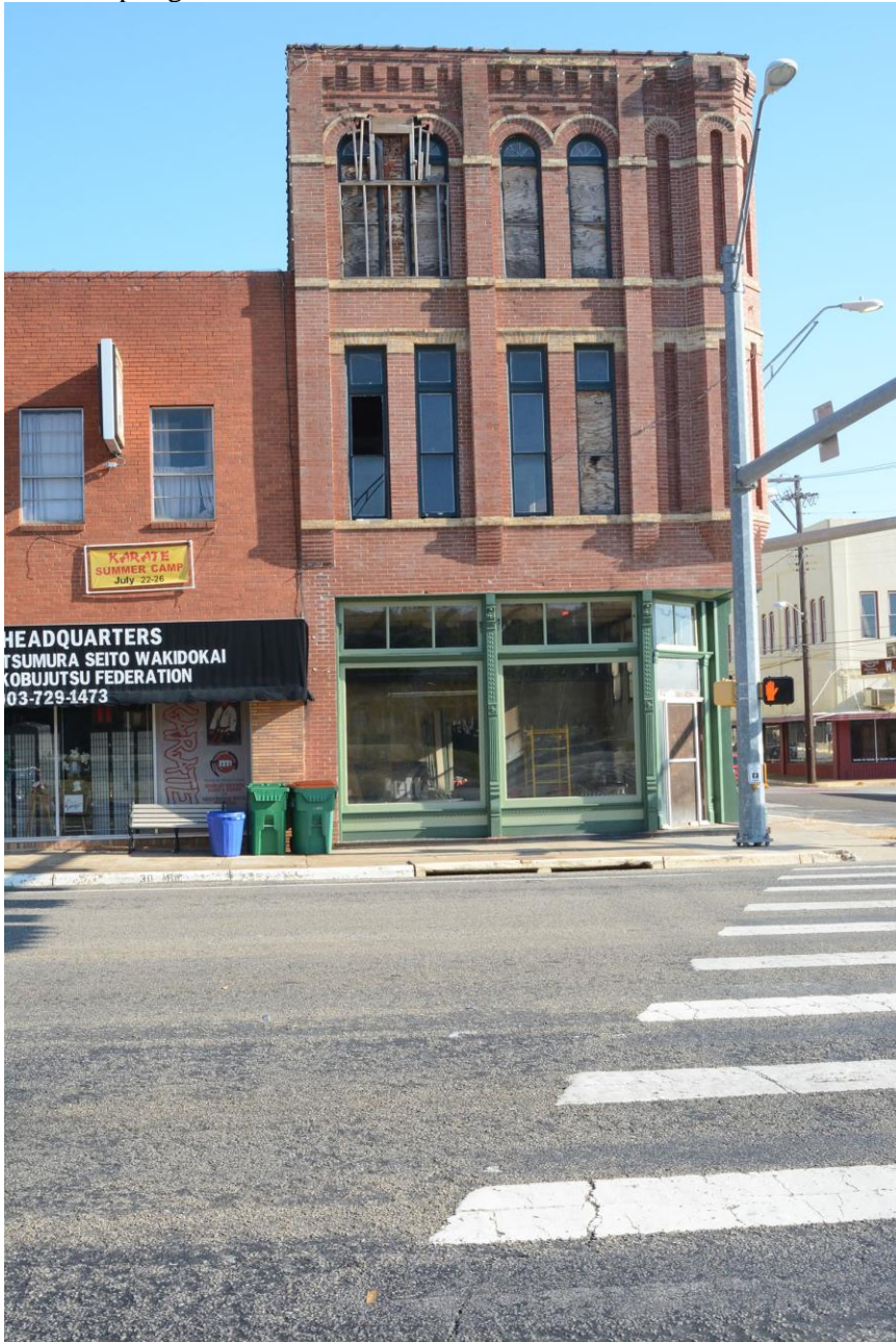
Photo 8 101 W. Spring Street
