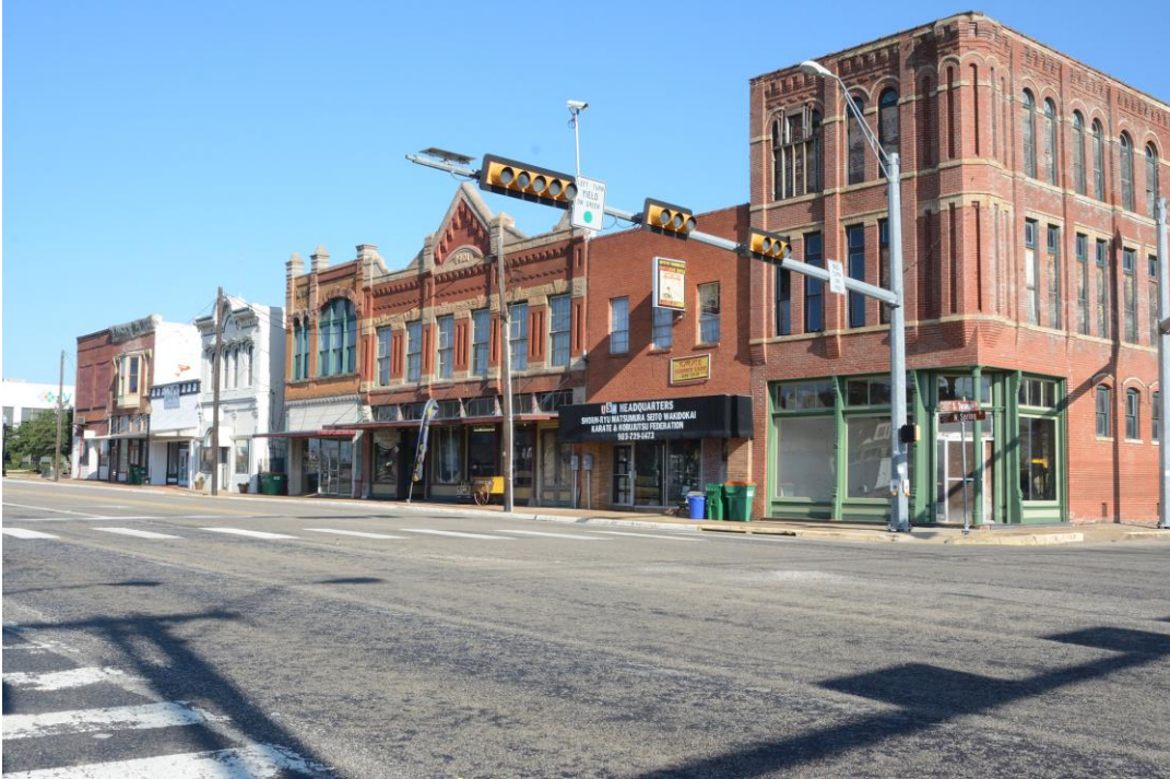
Photo 40 North Side 100 block W. Spring Street
