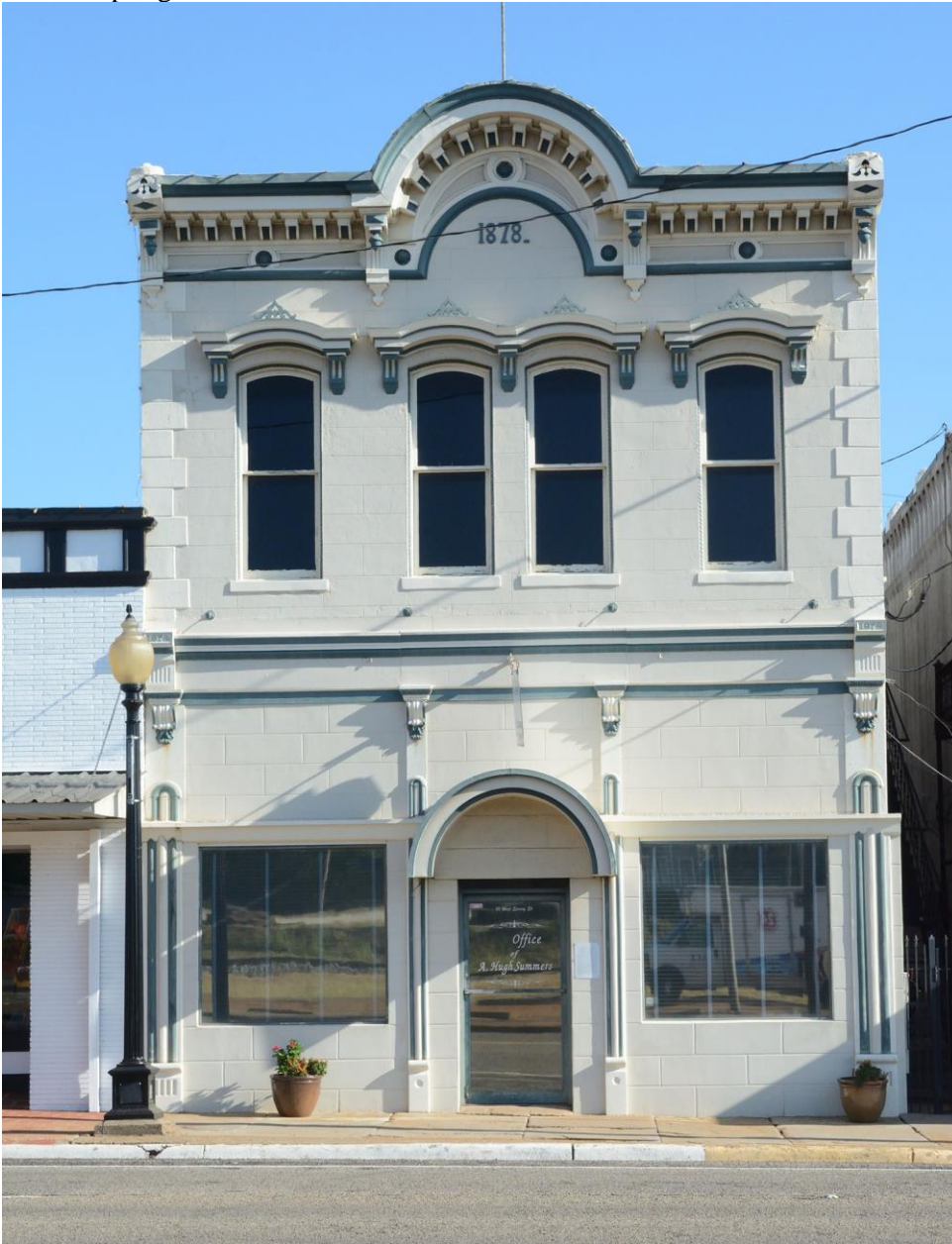
Photo 18 111 W. Spring Street
