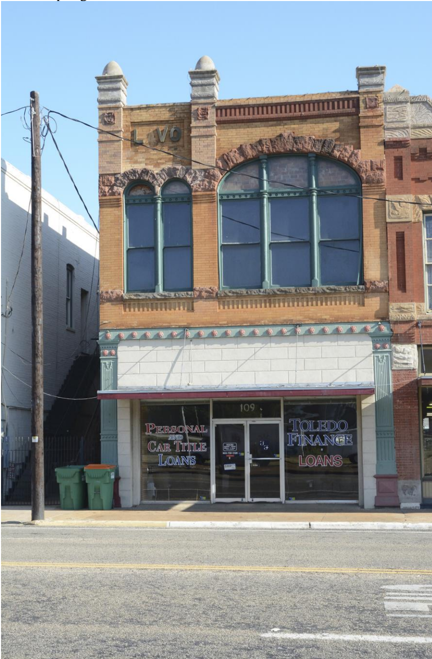
Photo 5 109 W. Spring Street
