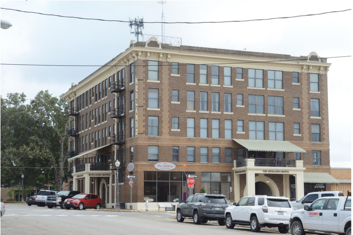
Photo 7 400 N. Queen Street
