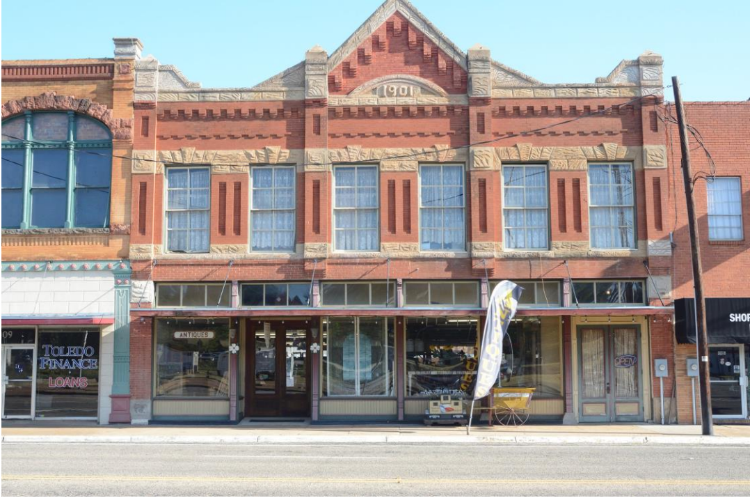
Photo 2 105-107 W. Spring Street
