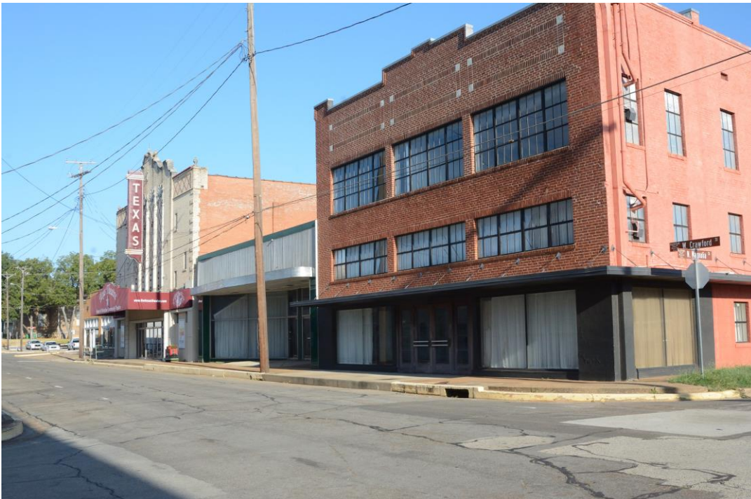
Photo 41 North Side 200 block W. Crawford Street
